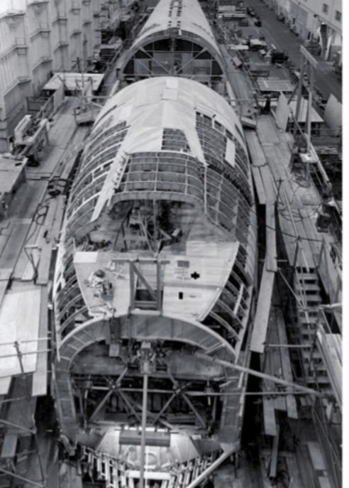
Seen here as it was being constructed, the H-4 was the largest airplane of its time. Unfortunately for Howard Hughes, the times were already passing it by, leading to controversy in Washington. The airplane's wooden structure also led to the popular sobriquet of "Spruce Goose," a name Hughes hated. In fact, the airplane was largely made of birch.
