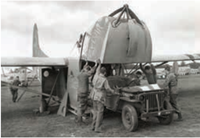
The CG-4A glider's adaptable cargo hold could be configured to carry heavy materiel like jeeps (left), a strapped-down howitzer and its crew of five (right), or more than a dozen soldiers and their gear.
